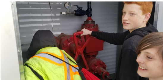
Conner at the wellhead of a geothermal pipe filled with water going over a kilometer down to get heated up. An example of a renewable energy source.
